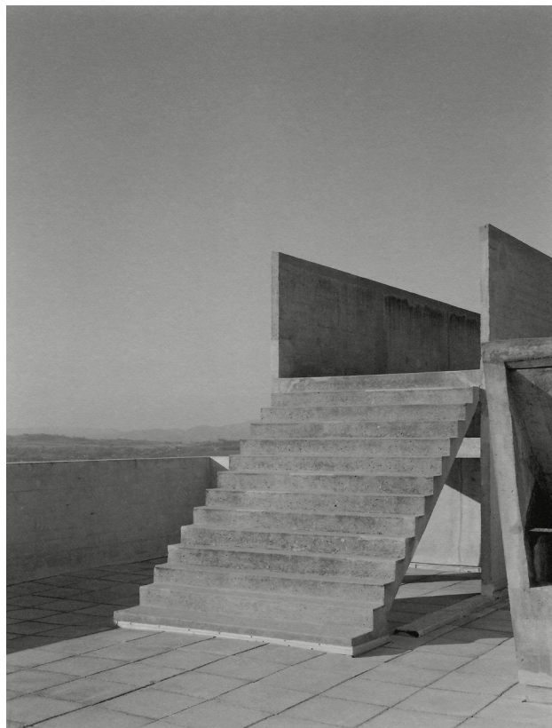
Jens Knigge, Couvent de La Tourette Stairway Roof Garden Architectures series ,
